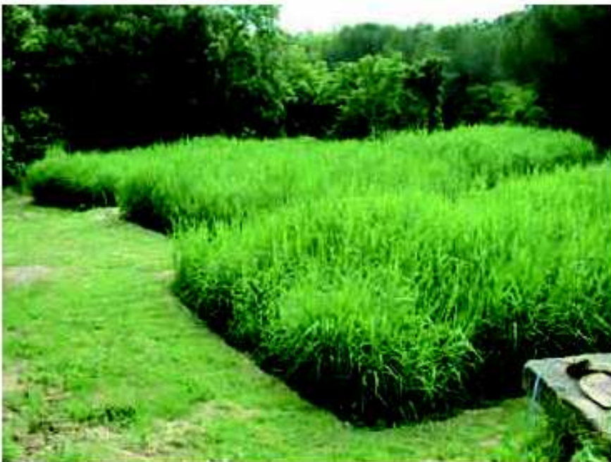
Figure 2: Constructed wetland of a winery, Italy
